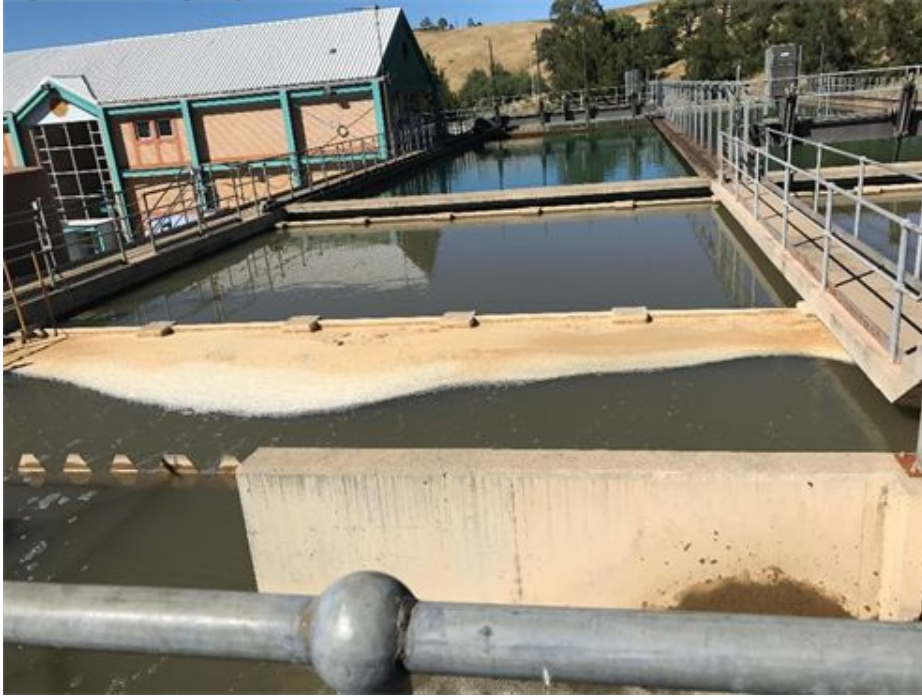
Figure 13-3 Jugiong Water Treatment Plant - Clarification
